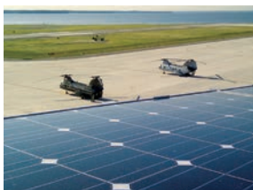
USMC, Quantico, 160kW hangar rooftop
