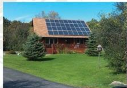
9.5 Kilowatt roof mounted system
