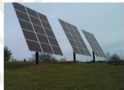
12 Kilowatt pole mounted system
